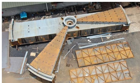
TYPE OF JOB - Tri-Sector Plate Assembly Industry – Power Plant HEIGHT AND WIDTH – 2.5 M Height and 16 Meter length, 4 meter width in dismantled condition WEIGHT – 60 MT approx.
